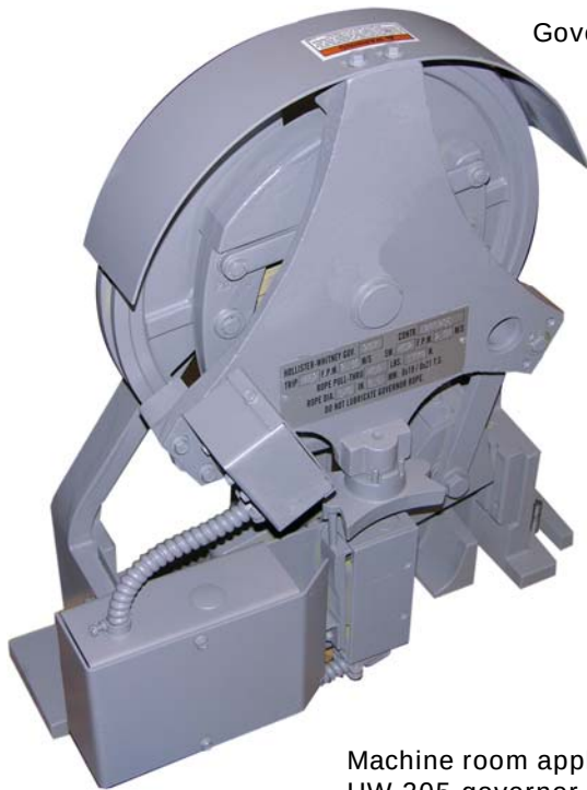
Figure 3.30 Governor Components
